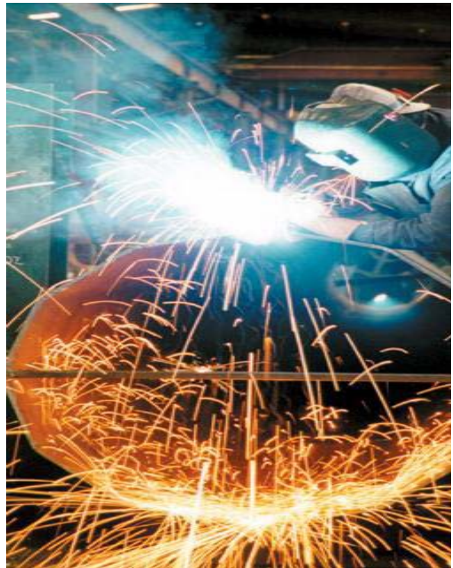
Fig . 8 : Welding of Steel Pole Vangs/ Accessories
