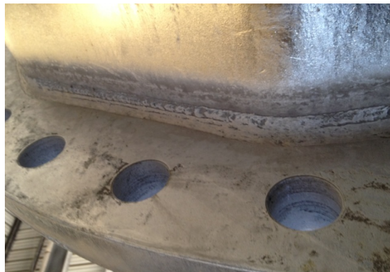
Fig . 16: Ready for Toe Crack Inspection
