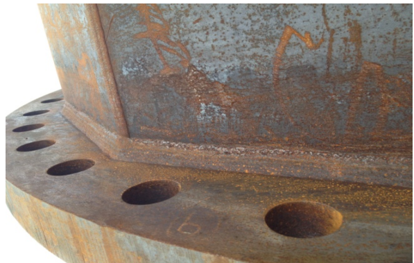
Fig . 12: Inspection of bolt holes & welding
