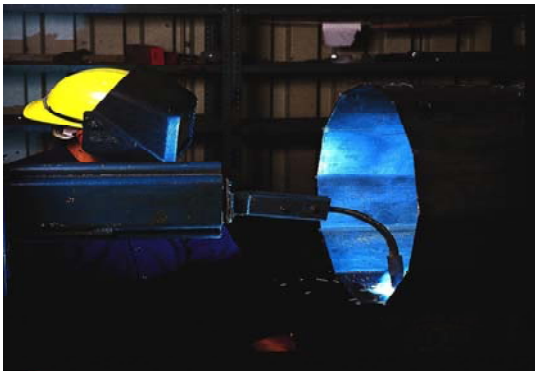
Fig . 7: Seam welding steel pole
