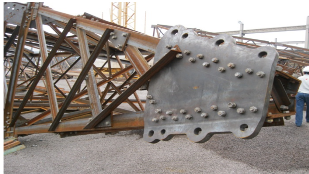
Fig. 27: Proof-of-fit of upper tower body
