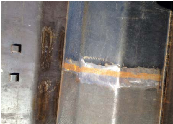
Fig . 11 : Inspection of pole weld and repair .
